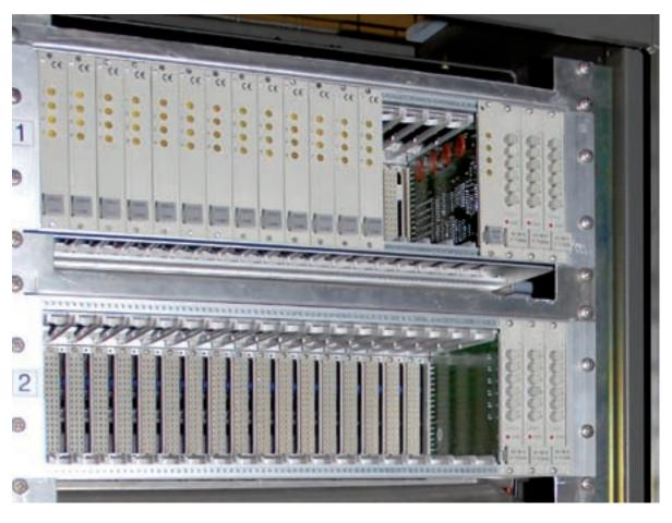
More space: **BP Lingen is** replacing more and more old 19inch temperature transducers with **DIN** rail devices from Turck
