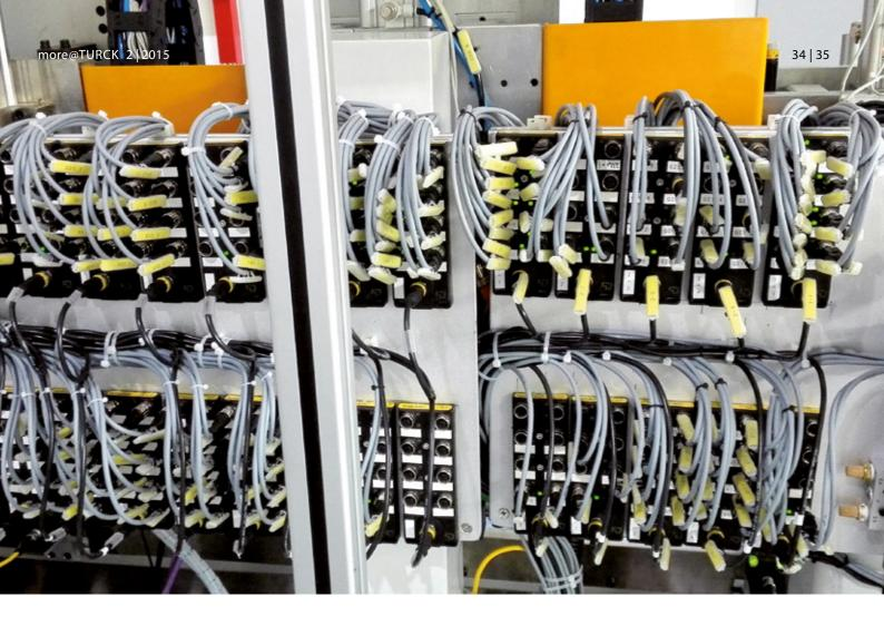
effect on the overall cost. Many cables for the passive junctions would have had to be prepared manually and then connected again to the I/O modules in the control cabinet. Commissioning would have been particularly prone to errors as well as being time consuming. The solution would also have been very expensive and difficult to maintain.
