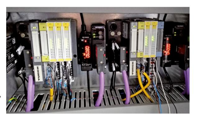
Besides hundreds of switching signals, two BL20 gateways also bring signals from RFID read/write heads and analog signals to the PLC
